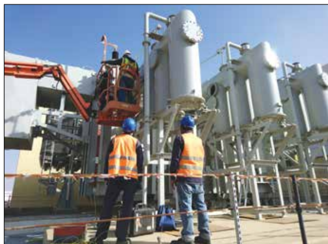
One of Kanoo's services is power TR testing
