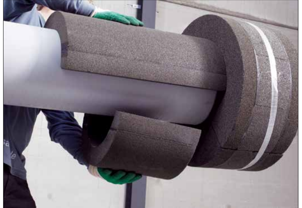
Prefabricated FOAMGLAS® impermeable insulation being installed
