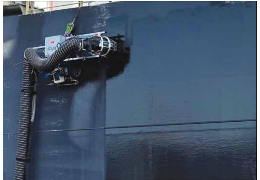
The 10Q robot is redefining industrial coating
