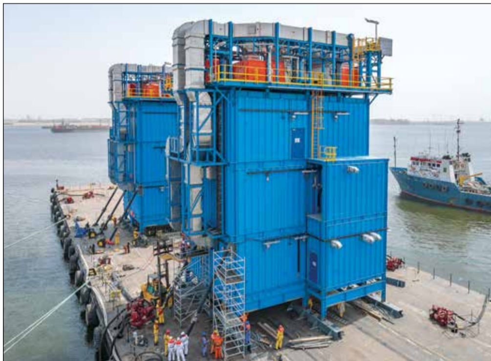
Specialist Services manufactures customised local equipment rooms and technical buildings
