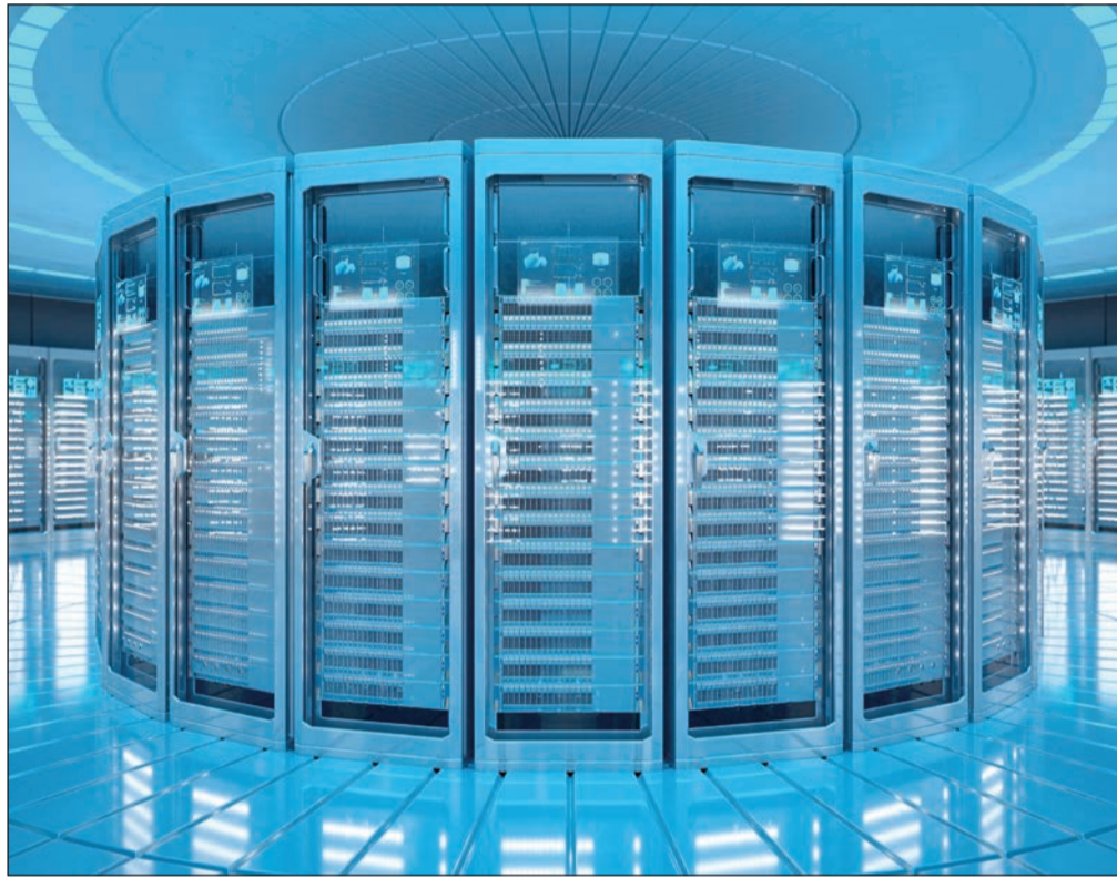
Data centres to drive growth in electricity demand
