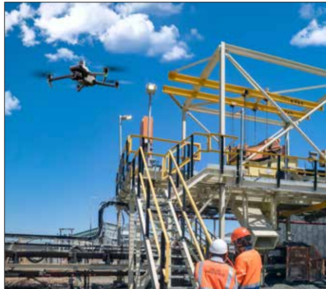
Drones make site monitoring efficient and precise
