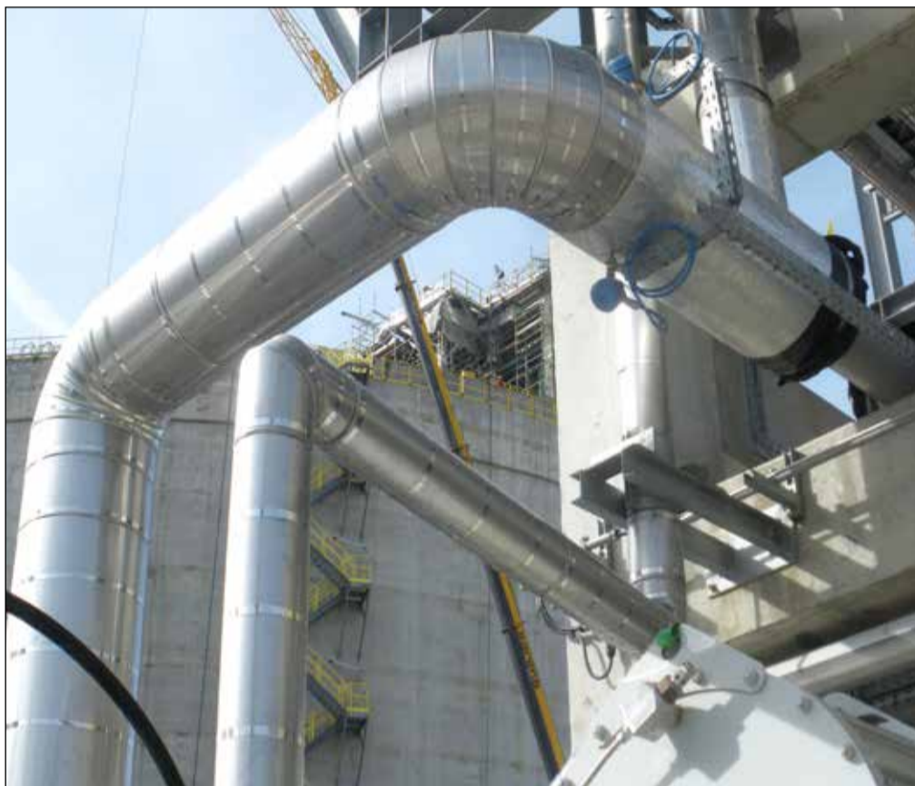
Cellular glass insulation can help protect joint seals and keep out moisture in LNG facilities
