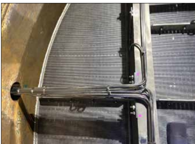
Sensors entering in the reactor and running on supporting beams
