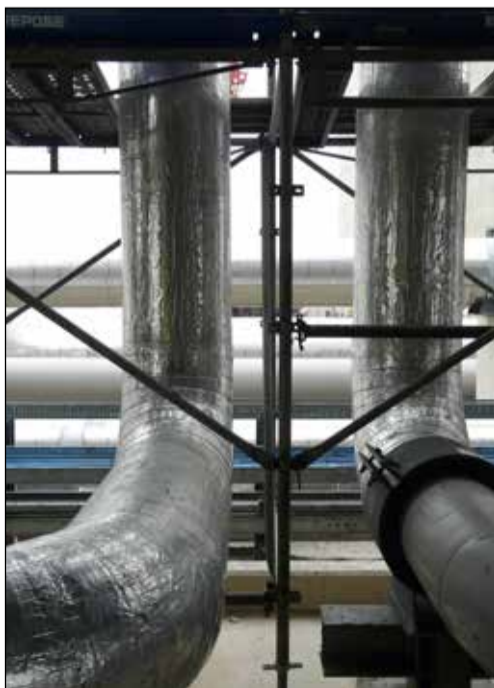
FOAMGLAS can reduce toxic smoke generation and help improve the safety of an LNG facility
