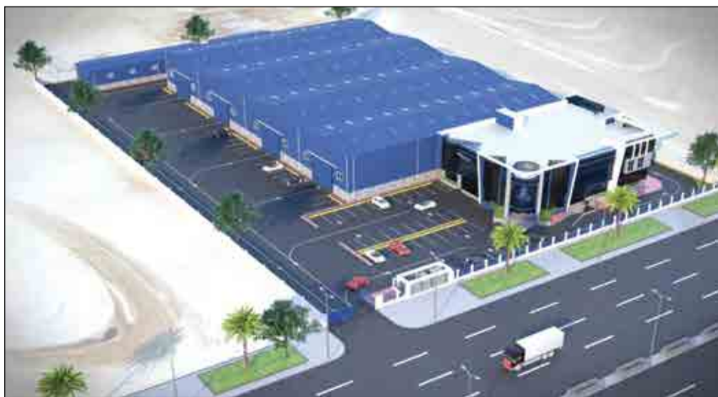
JAL International's fabrication facility in Jubail
