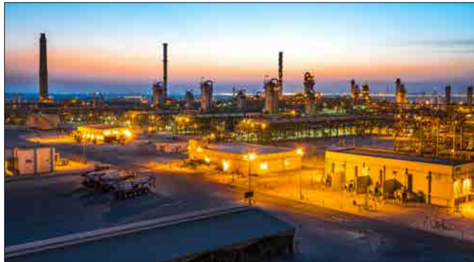
Jafurah has an estimated 229 trillion standard cu ft of raw gas
