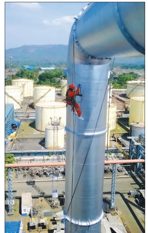
The rope access system in operation
