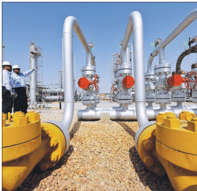
Bapco ... modernisation in progress
