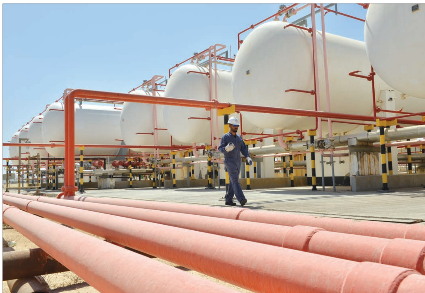
Banagas ... meeting the gas needs of Bahrain
