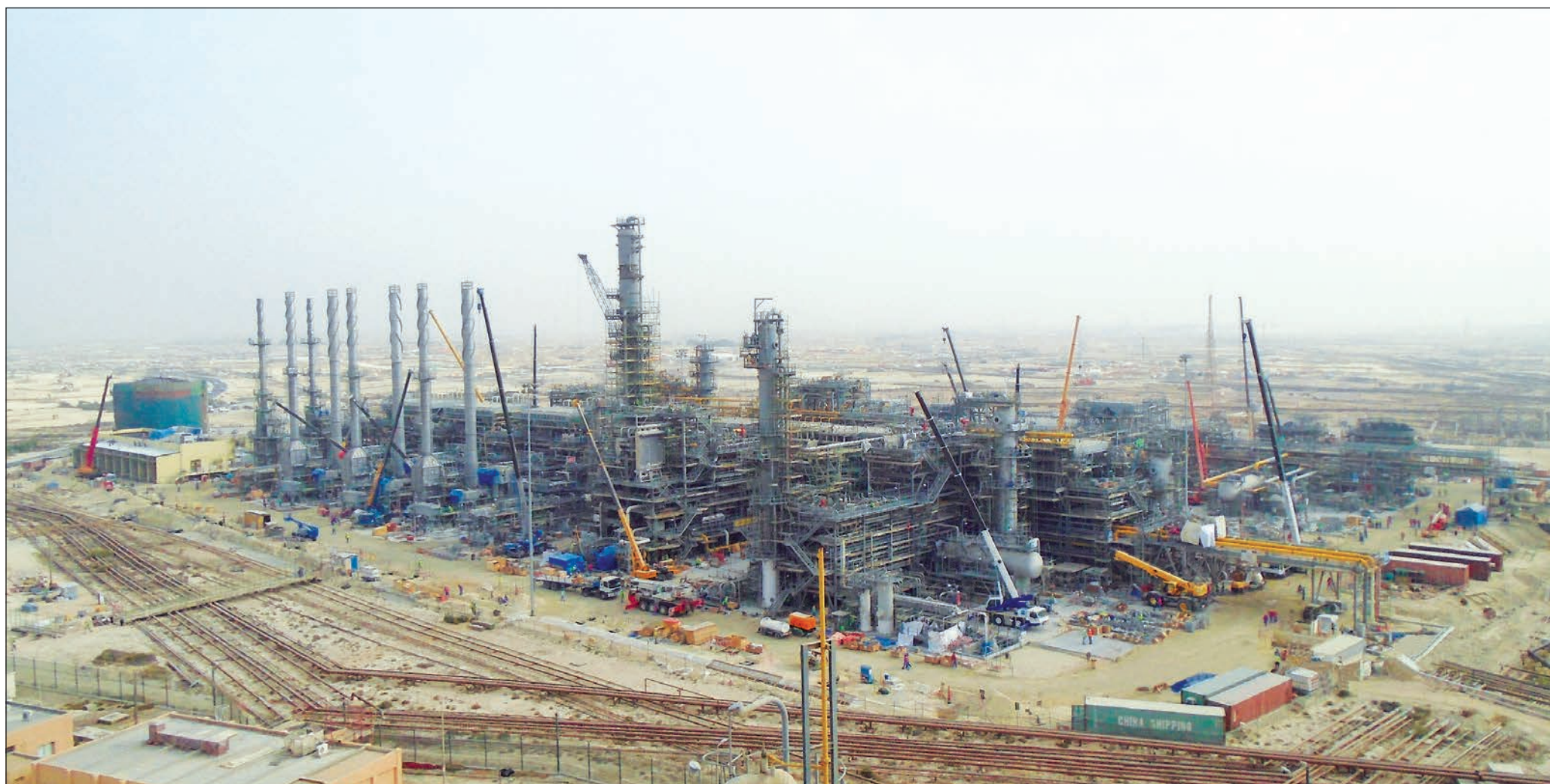
Banagas expansion in progress
