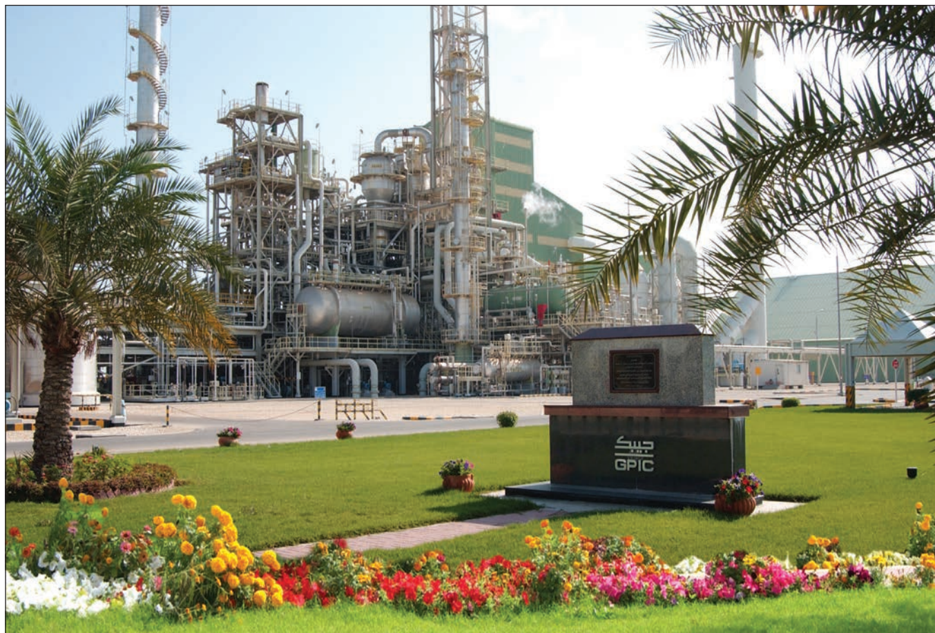
GPIC's urea plant
