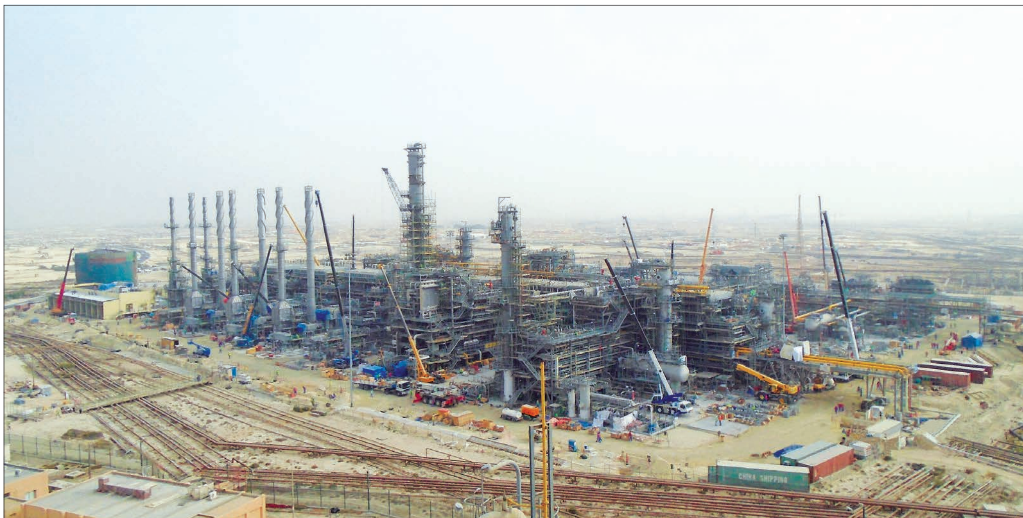
Banagas expansion in progress
