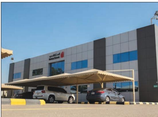
Inma Steel's new 65,000 sq m facility in Jubail
