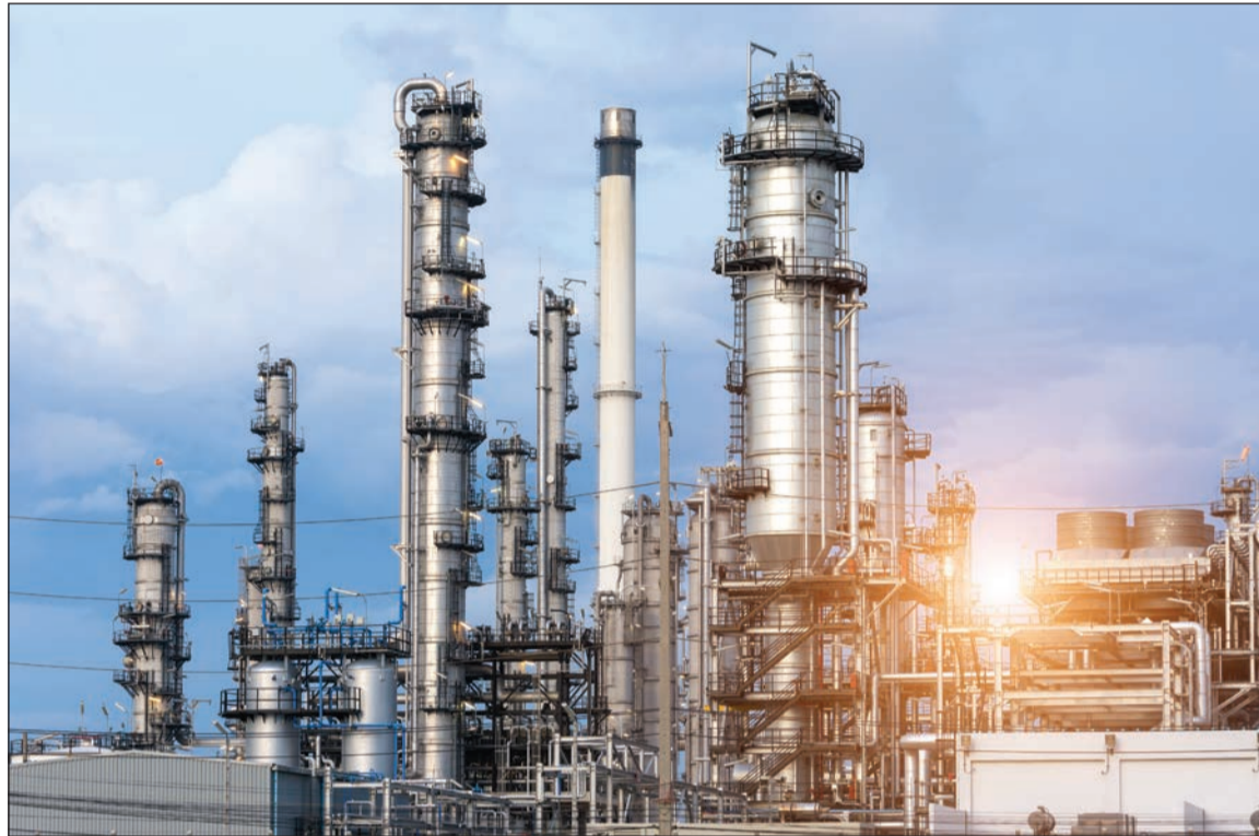
Refineries and petrochemical complexes can benefit from Sulzer GTC's GT-BTX technology
