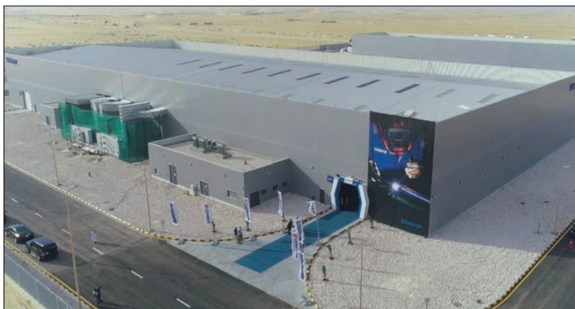
Schlumberger's facility at Spark ... world-class manufacturing
