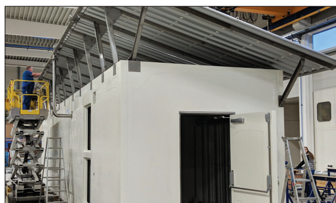
The shelter with its heat exchanger roof, sunshade, during construction at Intertec
