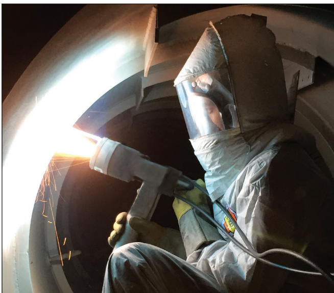
Application of HVTs on site
